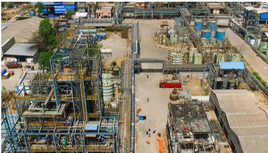
Photograph: Gujarat Fluorochemicals Limited Site Ranjit Nagar in Gujarat, © Green Power International Pvt. Ltd.
